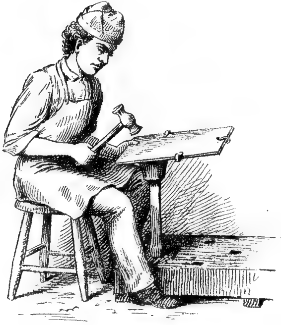
Fig. 19.—Planishing at the Block.
