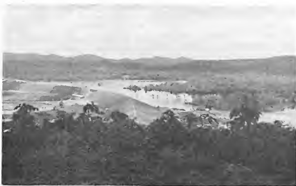
Fig. 1 — The barrage in the Suriname River at Ajobaka, with dead trees in the lake (June 1964).
