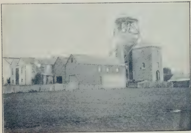
Plant at No. 9 Shaft of the Band and Albion Company. (Guiding Star line). (Looking north-east).
