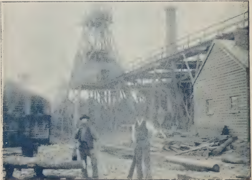
New Britannia Company's Plant, etc. (In Indicator belt of country). (Looking north-east).
