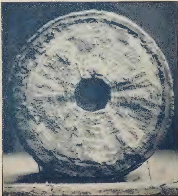
Section from inside of Pipe Connection between the Condenser and the Exhaust Tank. Principally earthy matter carried in mechanical suspension. Diameter, 8 inches.
