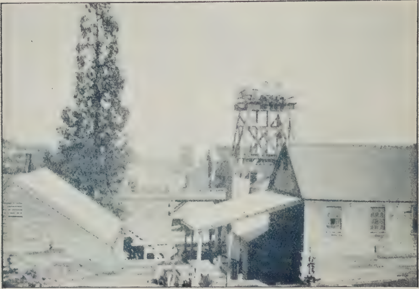
Sulieman Pasha Company's Plant, etc. On Sulieman Pasha line of lode, to the east of Indicator belt. (Looking south-east).
