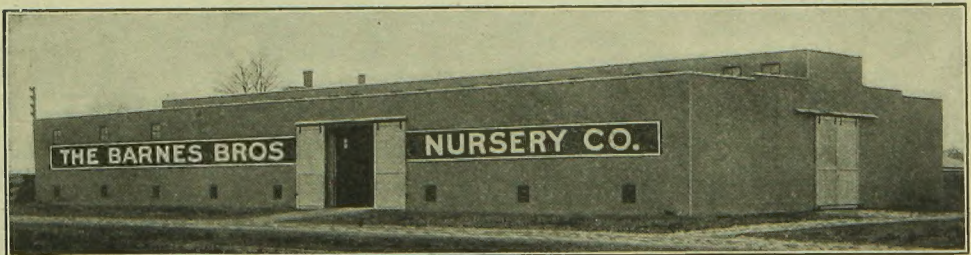
Our New Packing and Storage Building Looking from the Northwest
