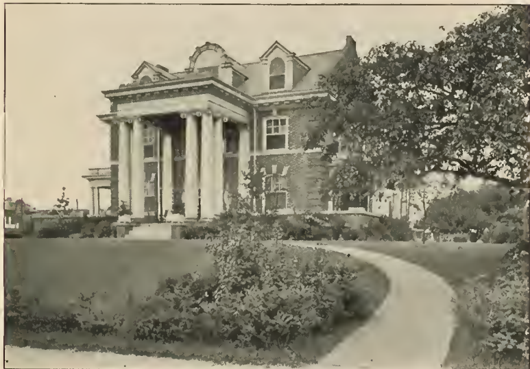
Residence of Mr. E. J. Stackpole, Harrisburg; the grounds planned and planted by us. Photographed first year after planting.
