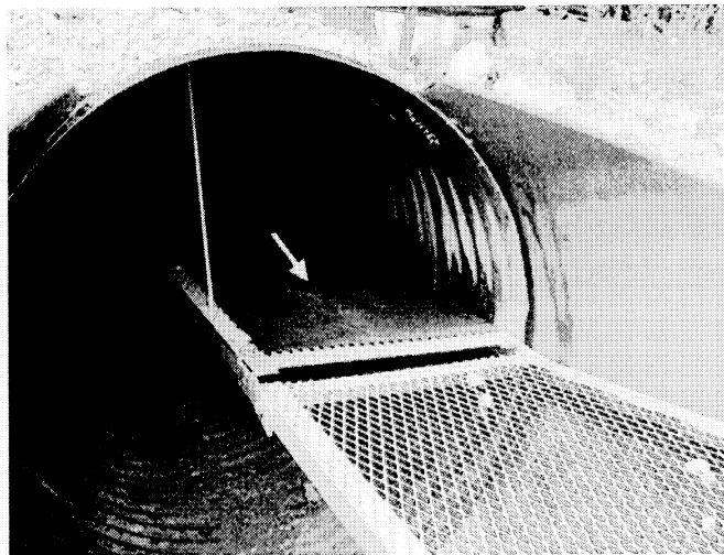
Figure 13. The shelf surface has been covered with heavy gauge plastic (truck bed liner material; yellow arrow) to provide a solid surface for smaller species.
