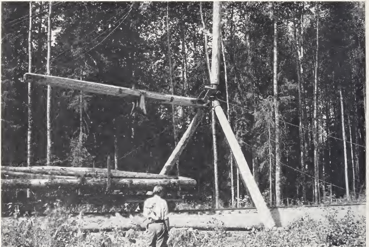
FIGURE 21.—Closeup view of tripod spar pole and loading boom.
