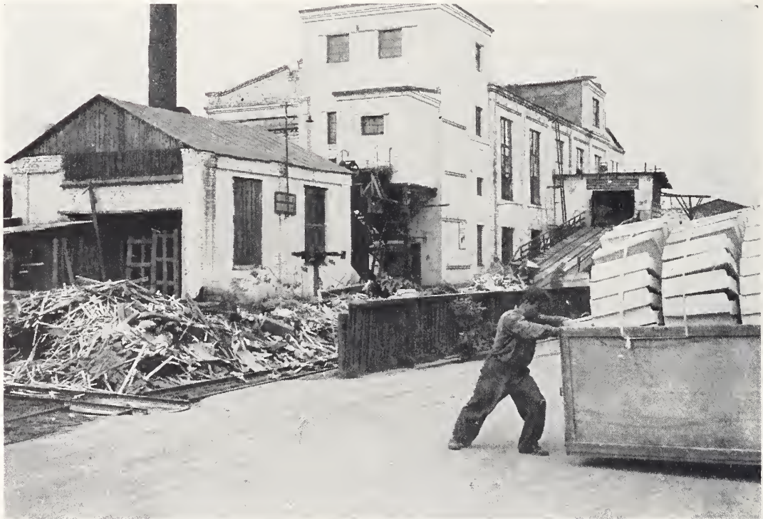
FIGURE 32.—Yard of the Bozhenko Furniture Plant. A high fire hazard exists due to poor housekeeping. No mechanical means are used for transporting furniture parts between the buildings.
