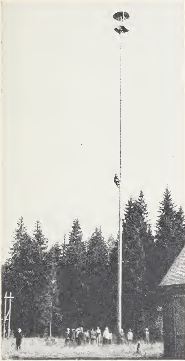
FIGURE 6.—Lookout mast about 115 feet in height on the Syversky Experimental Forest near Leningrad. The lookout climbs to the 4-foot-square "crow's nest" on handspikes. His ascent and descent are accelerated by a counterweight on one end of a wire rope that passes through a pulley at the top of the mast. The other end is attached to the climber's belt.
