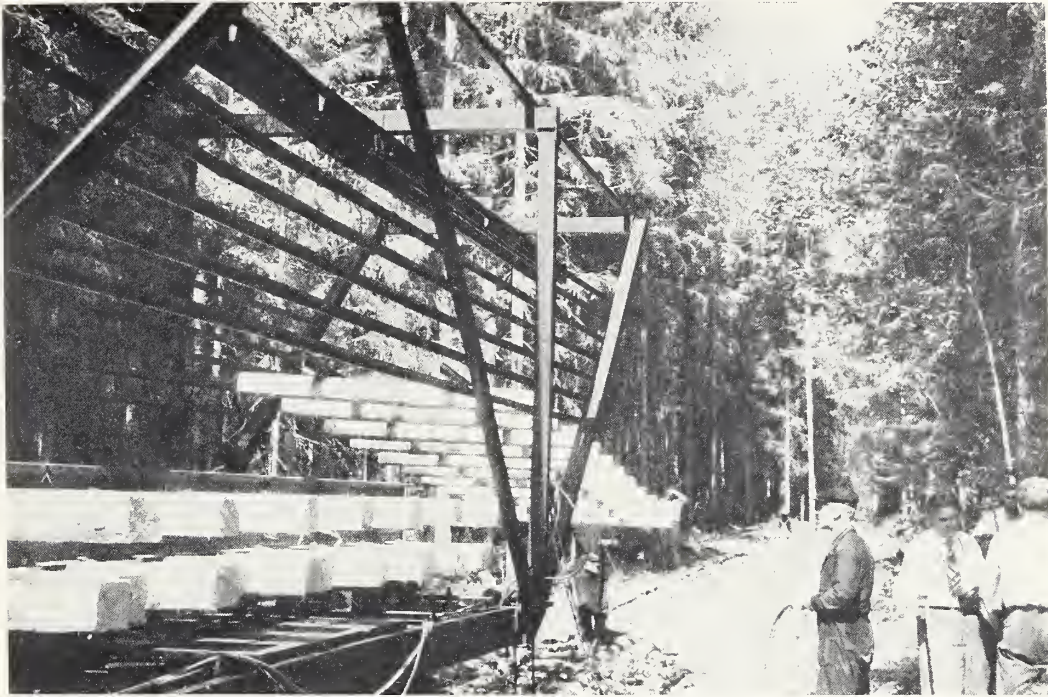
FIGURE 23.—Railroad track-laying machine.
