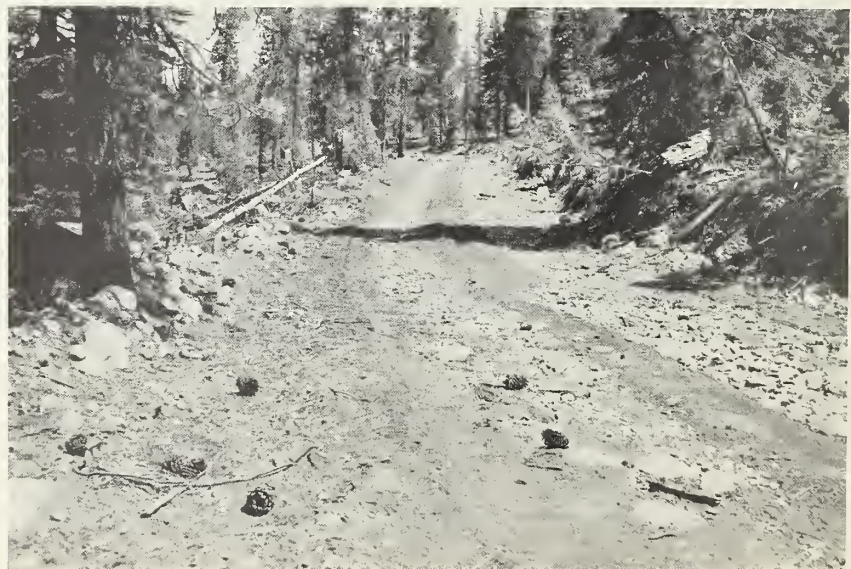
Abandoned temporary road showing severe erosion of the roadbed.
