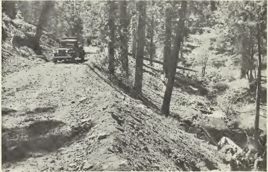
Temporary road properly located along a creek.
