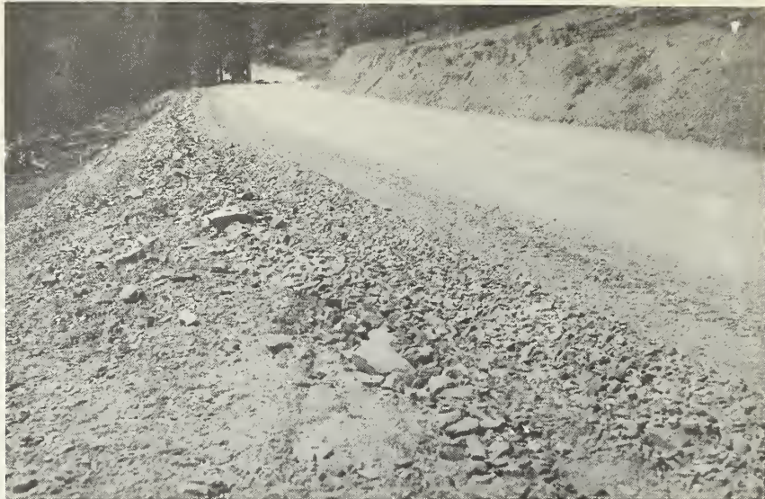
Main road on hillside location in rocky shale soil.
