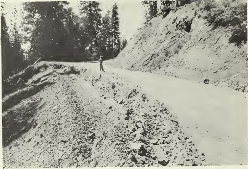
Main road in difficult location across wet slide area in serpentine-shale formation.
