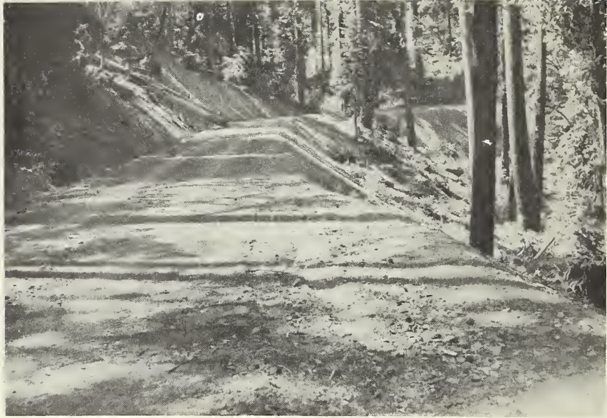
Secondary road on contour location in shale soil.
