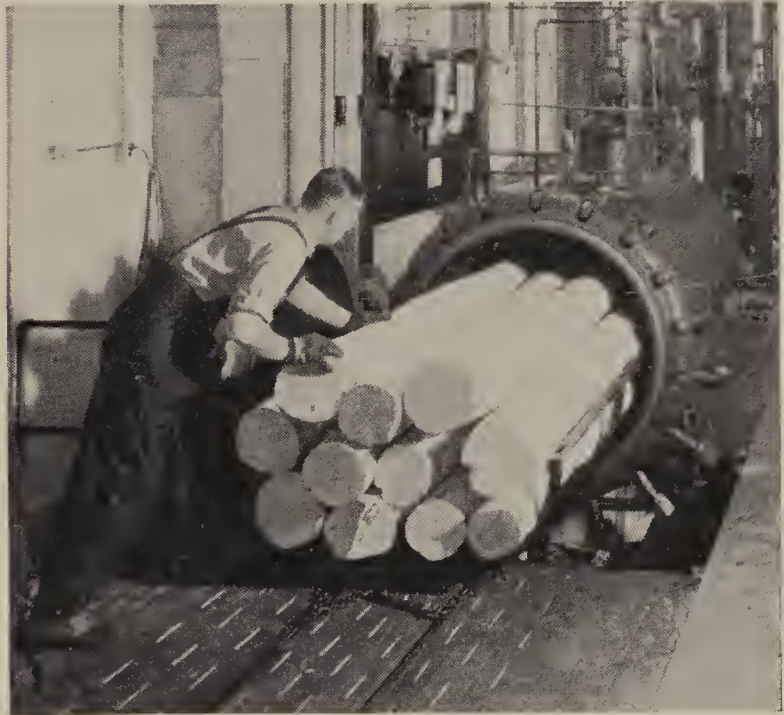
Experimental preservative treatments of wood at the Forest Products Laboratory are checked by subsequent service tests.
