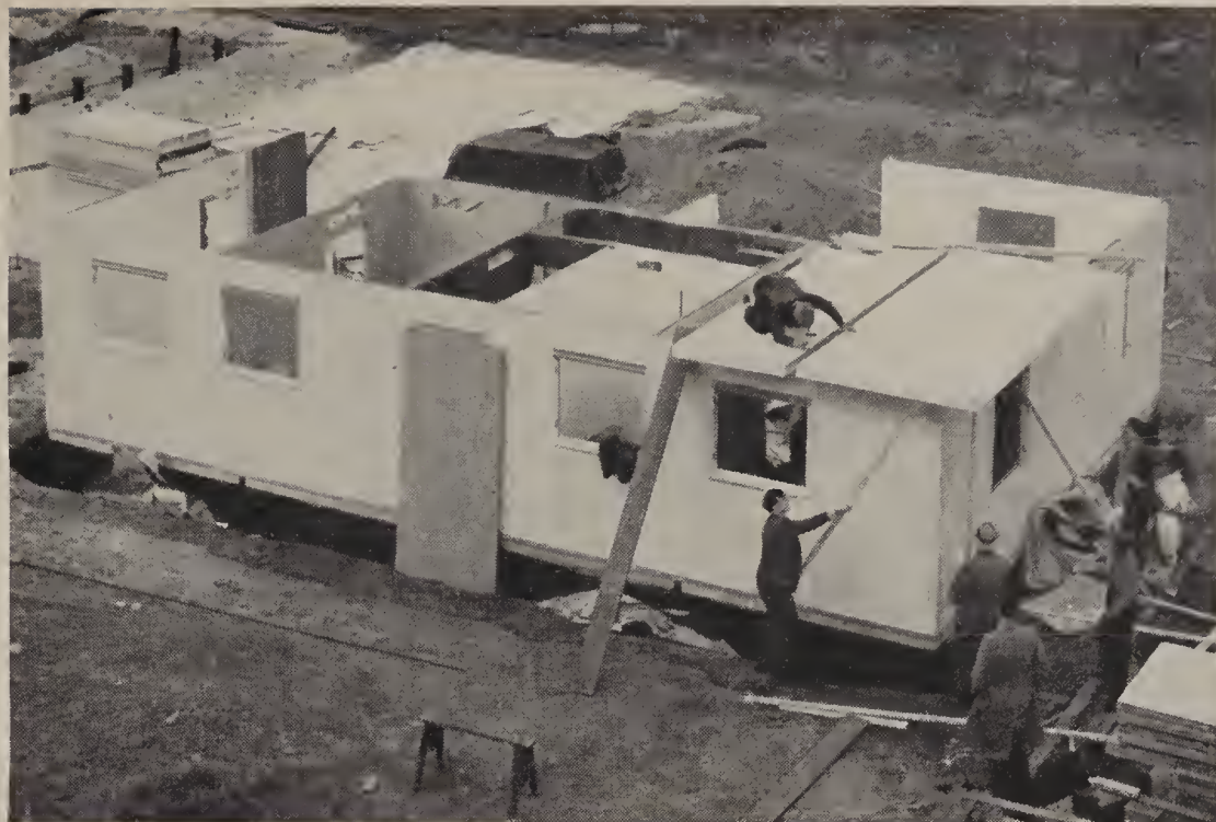
Erection of demonstration prefabricated house at Forest Products Laboratory.
