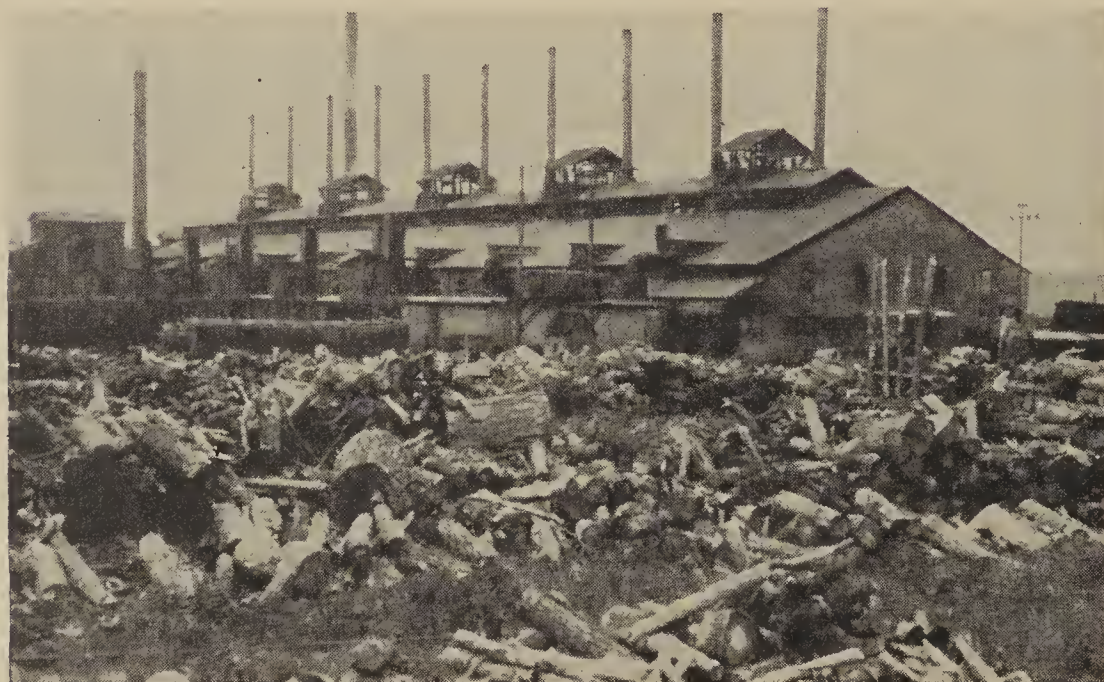
Wood distillation affords a use for cull trees, limbs, tops, and other material not suitable for lumber.
