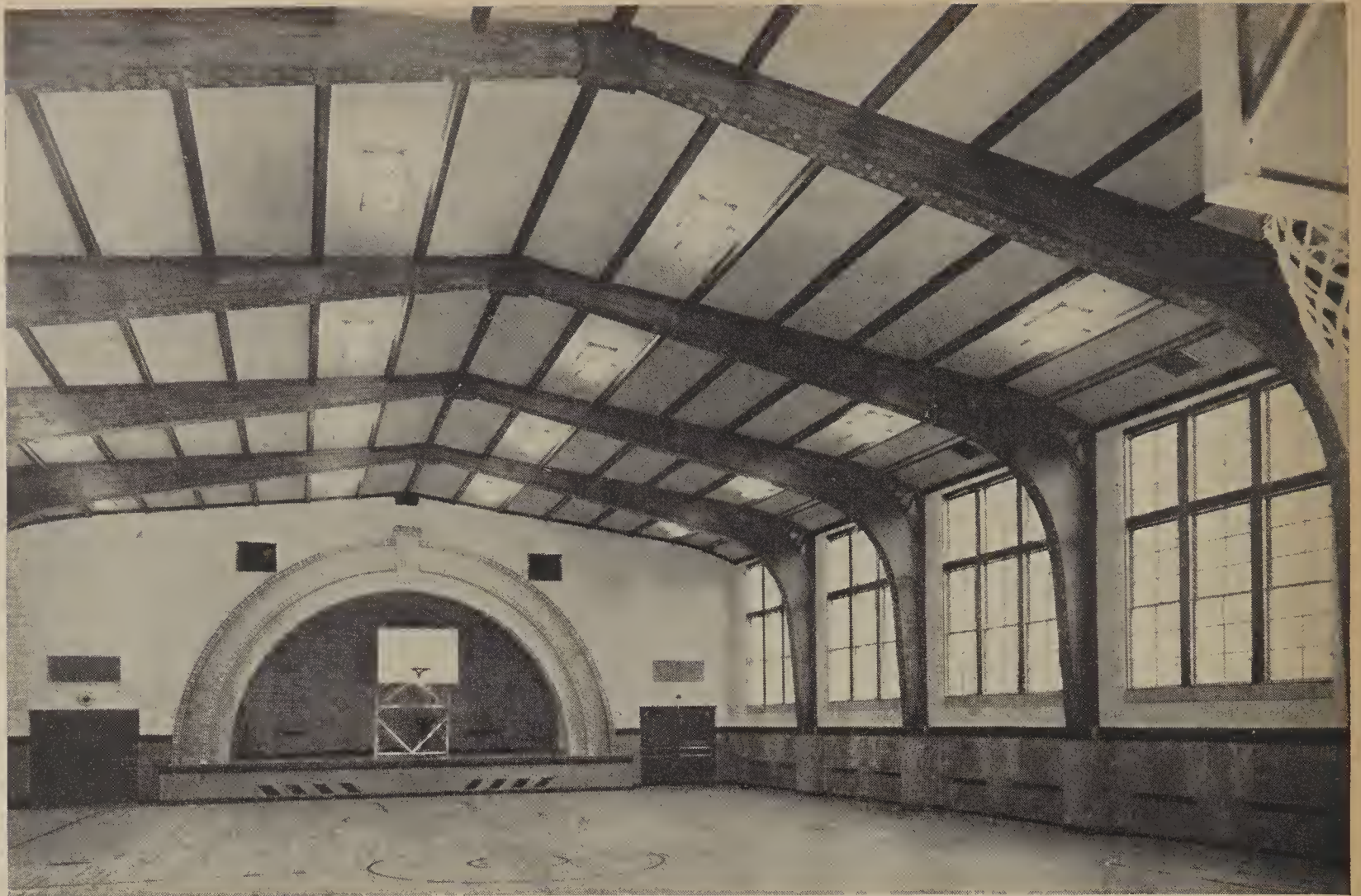
A high-school gymnasium framed with glued laminated wood arches.
