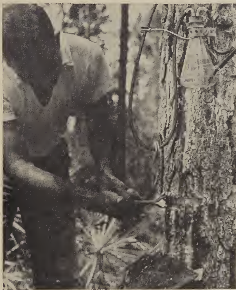
Narrow chipping lengthens the resin-producing life of the southern pines.
