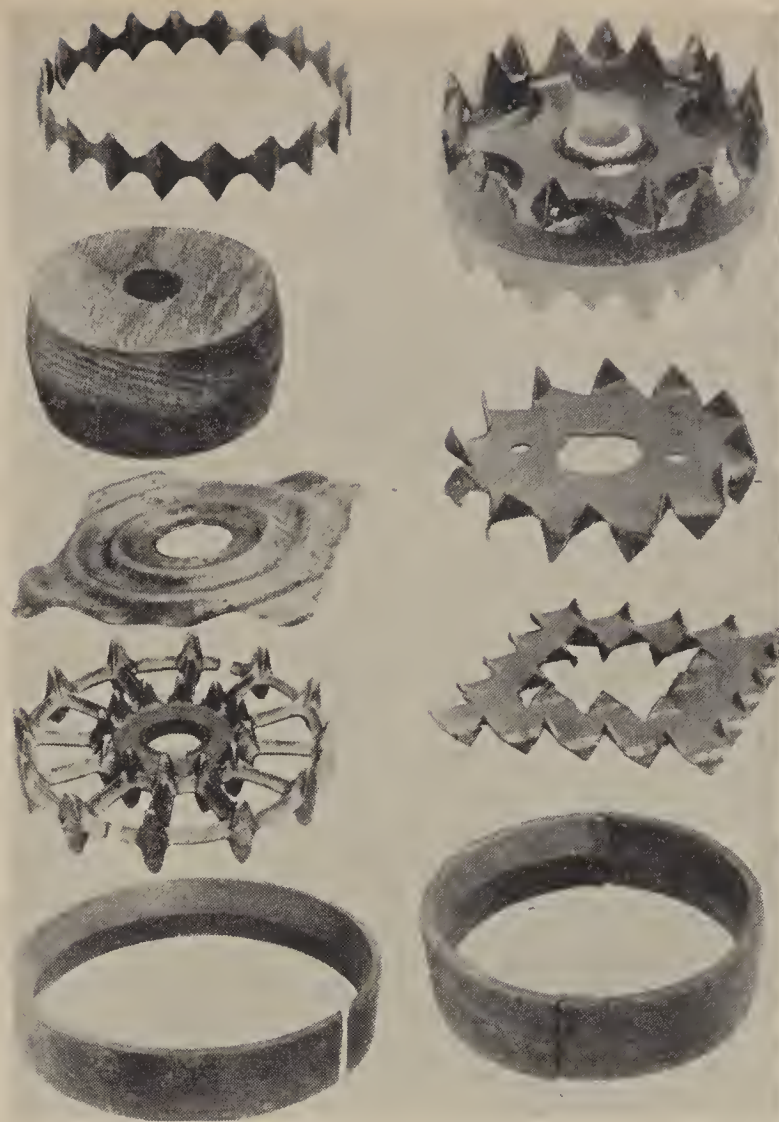
Types of modern timber connectors.
