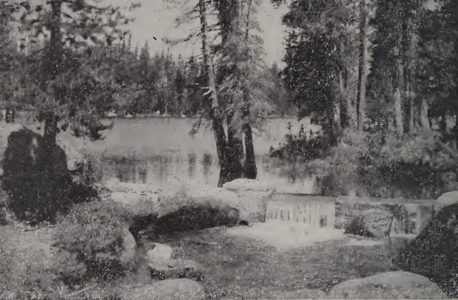
Small dam at outlet of lake maintains enough water in stream below to support fish life during the summer.
