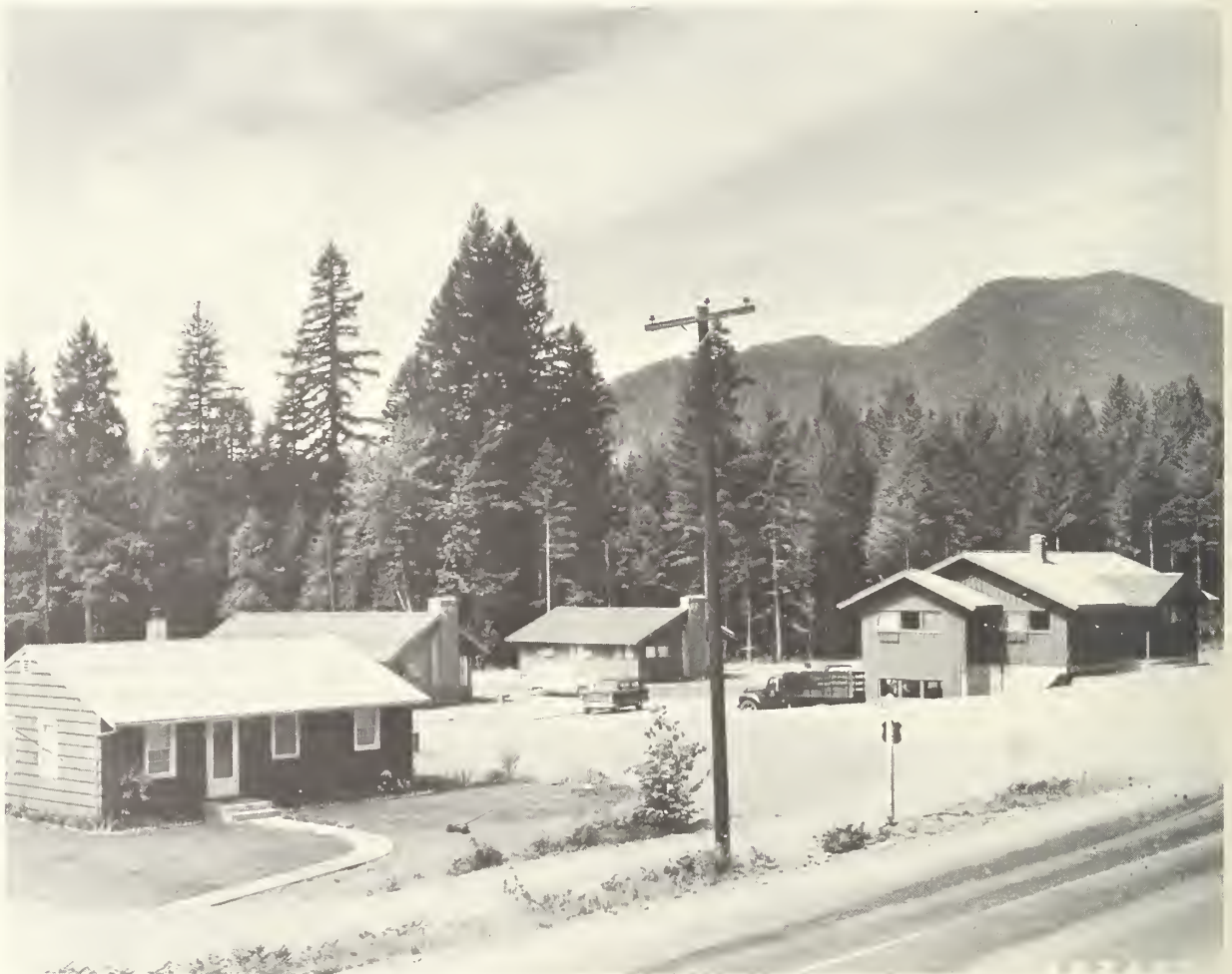
Adequate housing and service facilities for field personnel.
