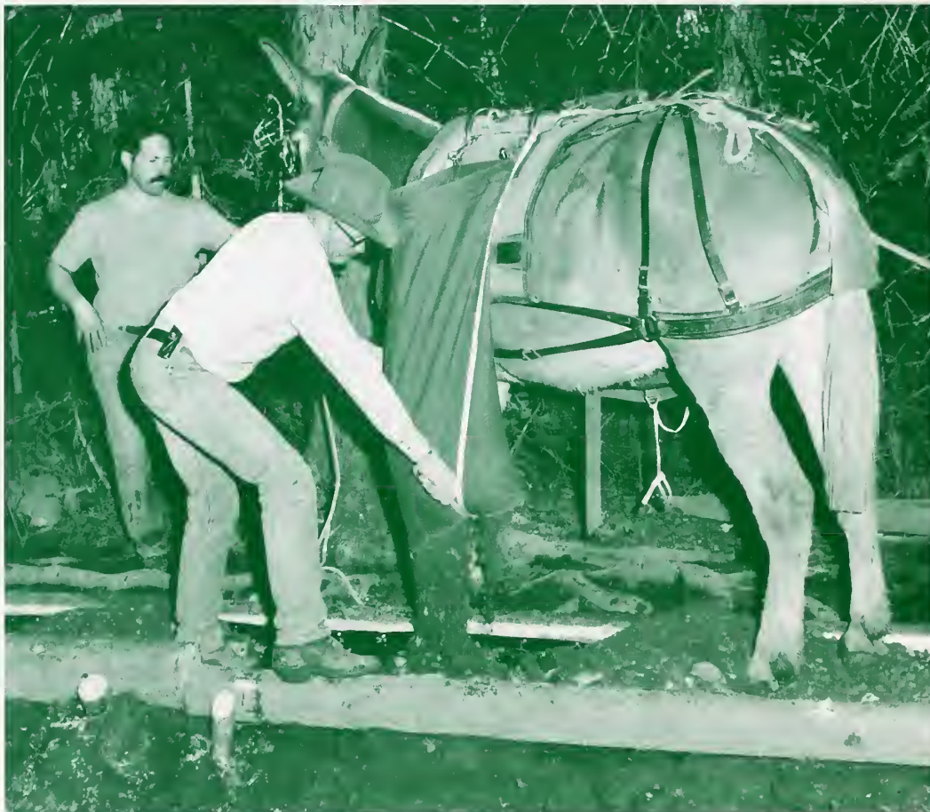
Figure 4.—Bags allow directing the flow of material under or away from the pack animal.
