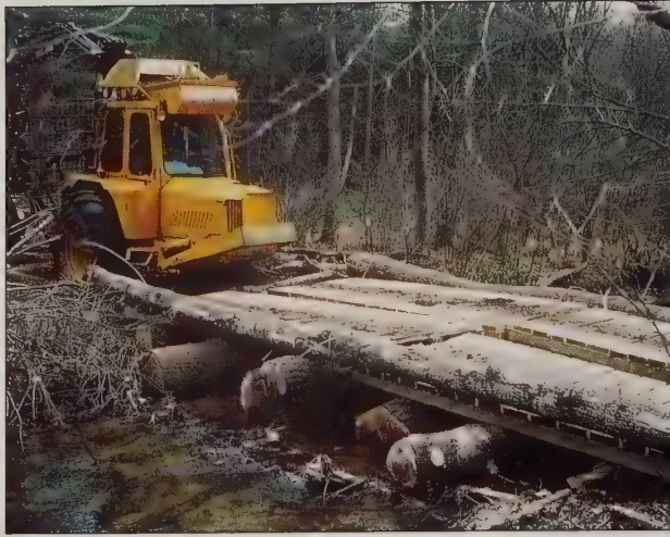
▲ These skidder ramps are lighter weight and will sometimes require logs for support.
