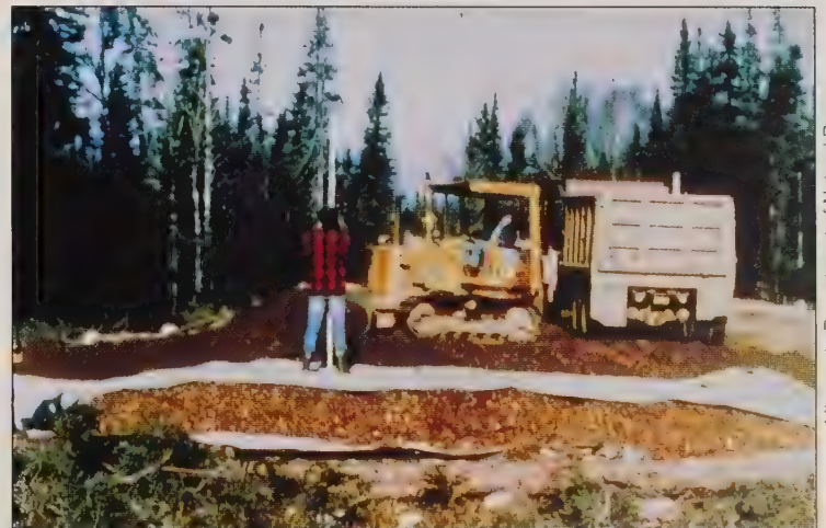
▲ Another layer of geotextile is placed on top of the chunkwood to prevent contamination and sealing of the porous layer. The gravel running surface is placed on top of the geotextile fabric.
