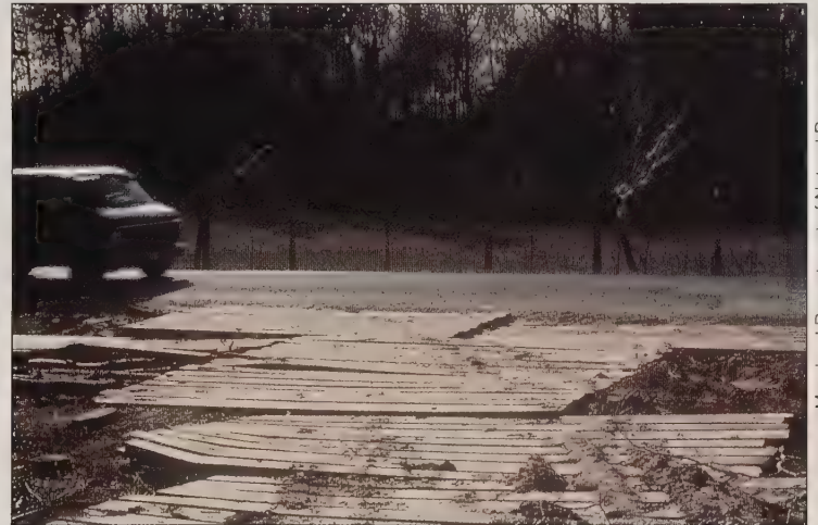
▲ Wooden mats can be used to provide mud-free highway approaches.
