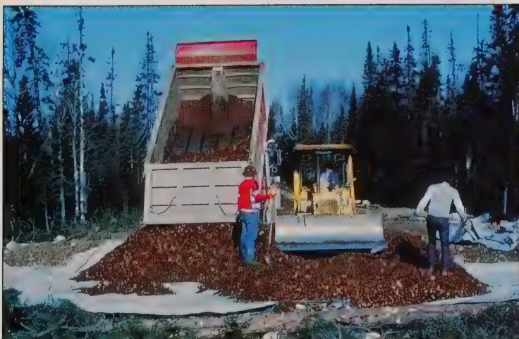
▲ Geotextile is then placed on top of the corduroy along with a layer of wood chunks to form the porous layer. Coarse gravel could be substituted.
