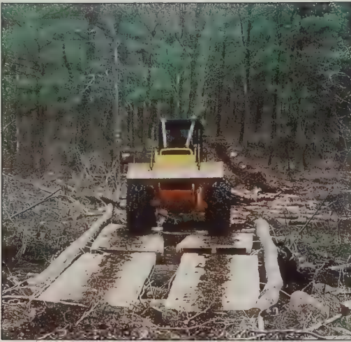
▲ Corduroy approaches help to control erosion and keep mud off the logs and out of the stream.
