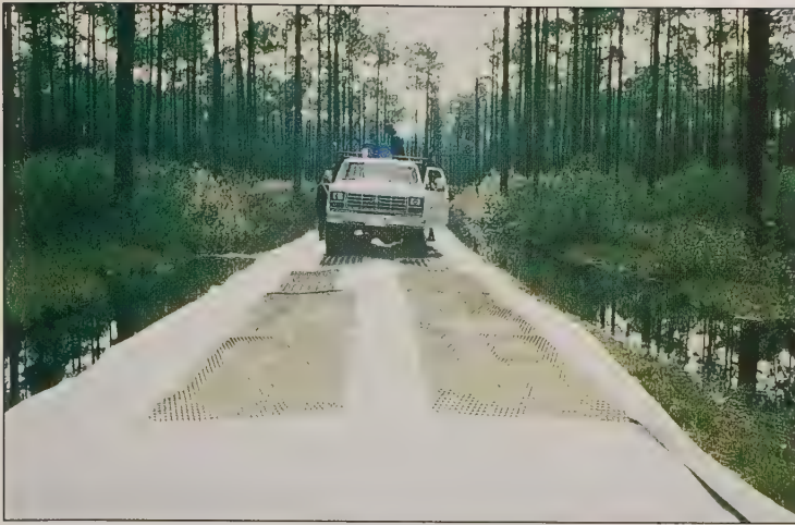
▲ Geotextile and expanded metal sheets are used to strengthen an existing road.
