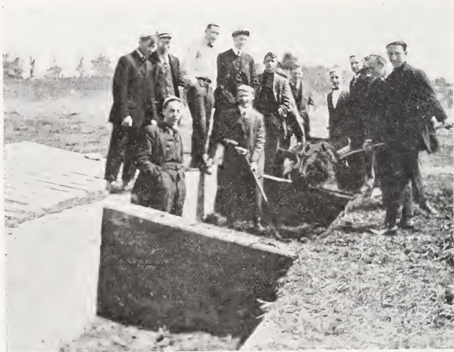
Fig. 18—Students filling a concrete hotbed pit
