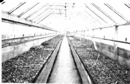
3. ONE OF our new mist propagation houses. Automatically controlled, maintains ideal growing conditions to produce healthy husky root systems.
