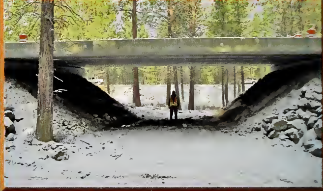
Shown while still under construction, the first wildlife underpass for the newly divided US 97 south of Bend will provide passage opportunities for all wildlife in the area when completed. This highway project incorporated many 'Green Highway' features, including wildlife crossing structures. (Image: Oregon DOT)
