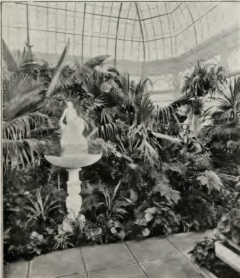
Interior of Palm House in above Range.
