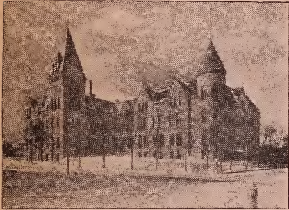
Central High School, Minneapolis, Minn.
