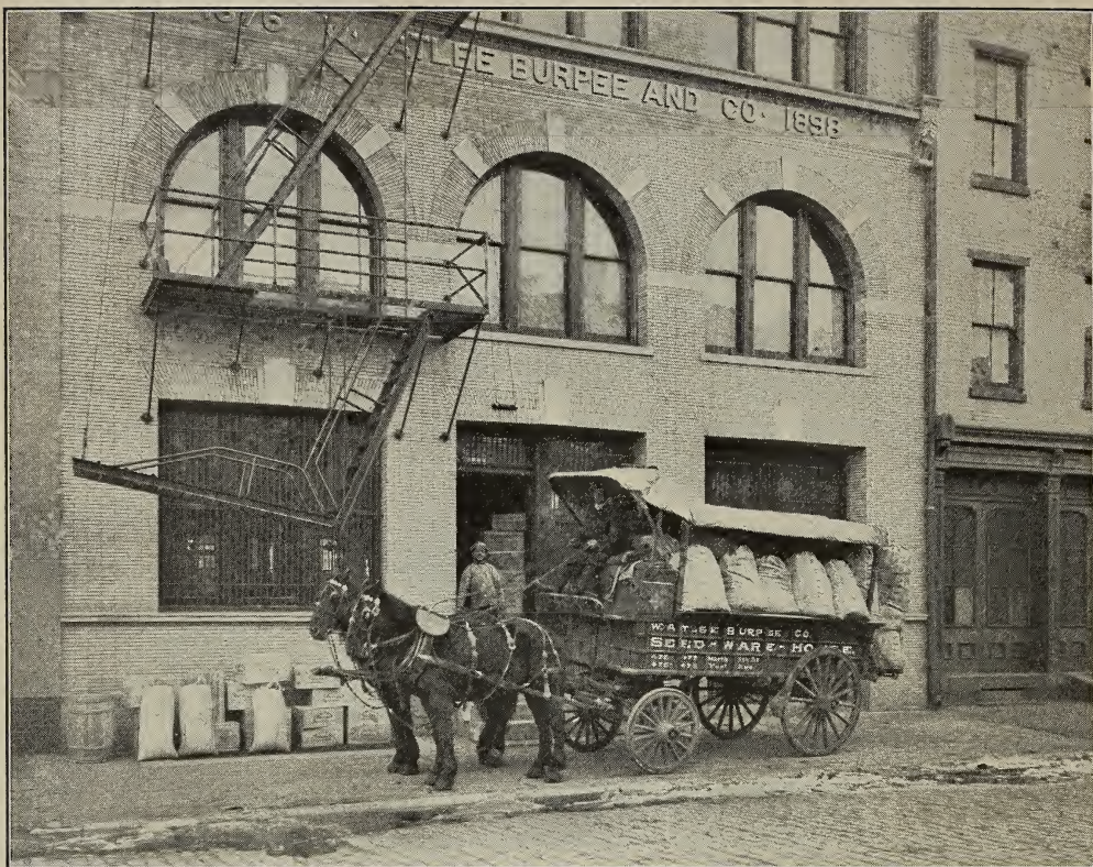
"READY FOR THE POST OFFICE,"—in front of the new Burpee Building.
