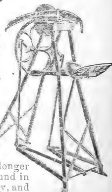
Adjustable Tool Grinding Rest.
