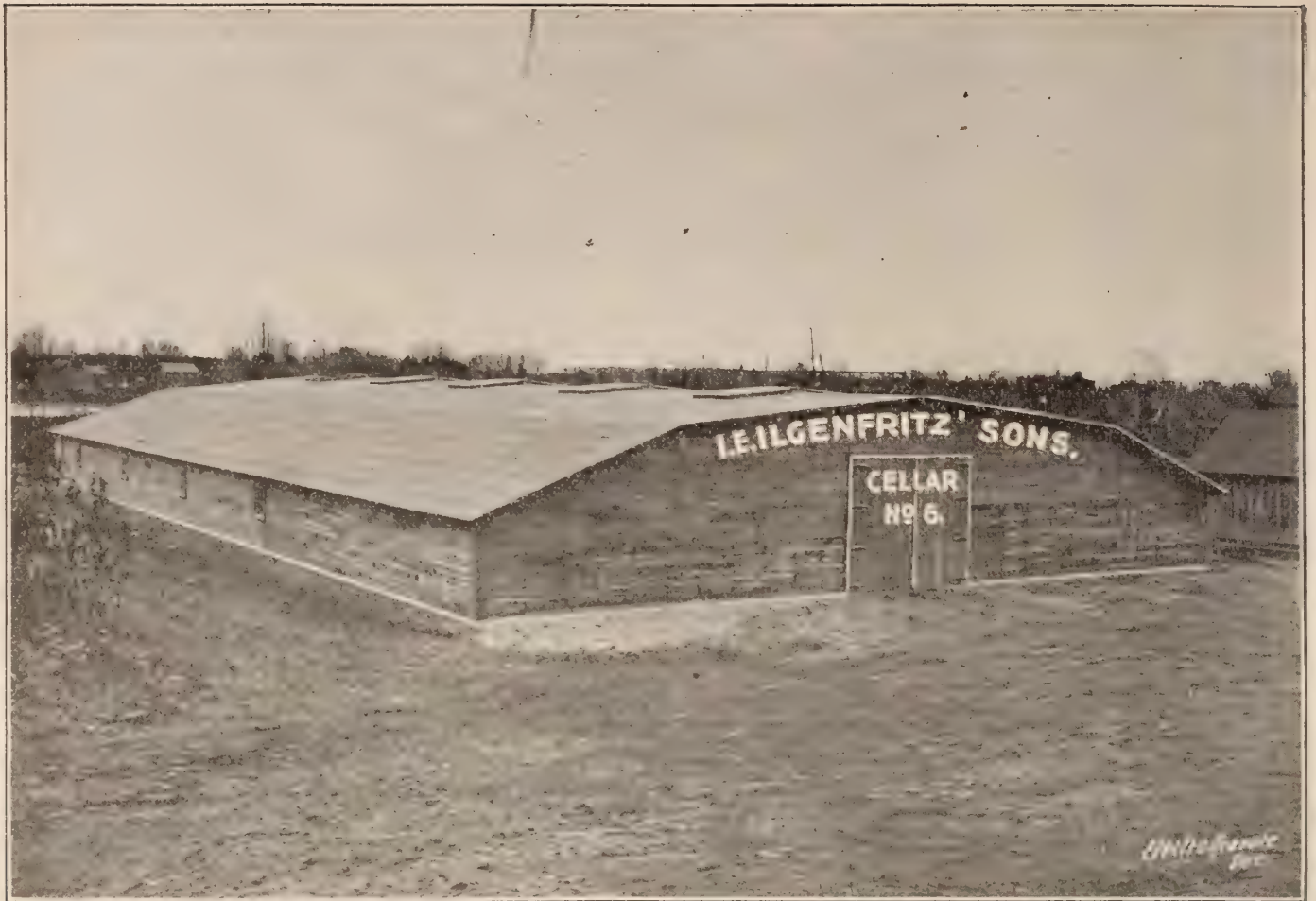
STORAGE CELLAR, NO. 6.
