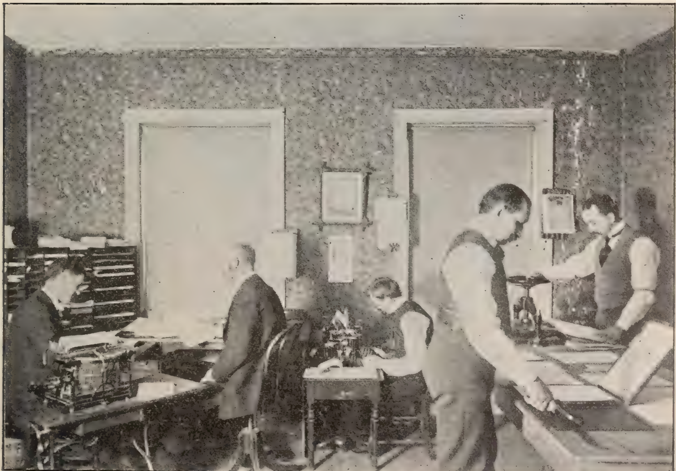
AGENCY DEPARTMENT ROOM—6
