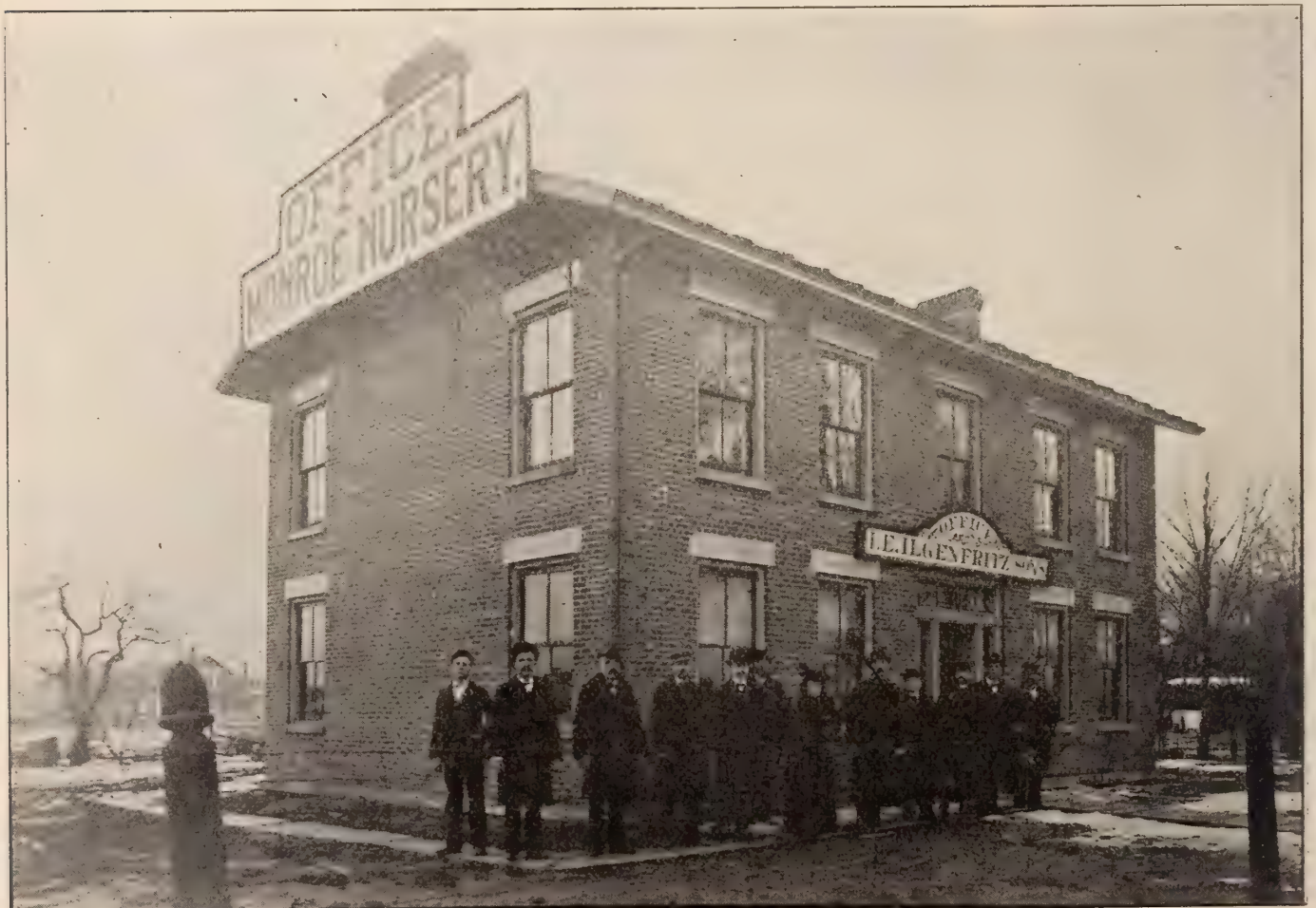
EXTERIOR OF OFFICE.
