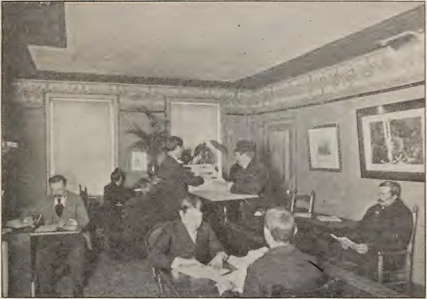
GENERAL OFFICE—ROOM I
