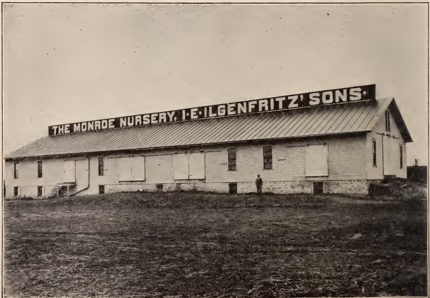
STORAGE CELLAR —NO. 2.
