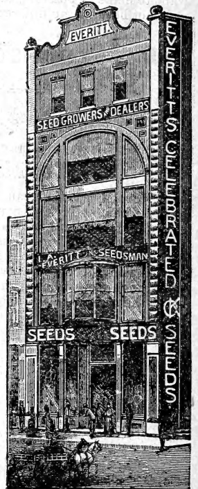
The Home of O. K. Seeds. The Building is Five Stories and Basement; 195 feet deep.
