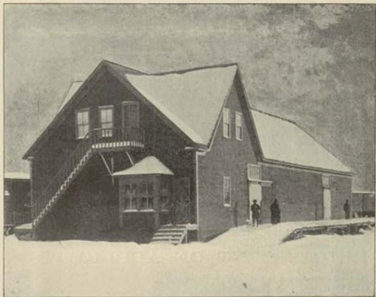
One of our Storage Houses at Presque Isle, 160x40 feet. Capacity 15,000 barrels.
