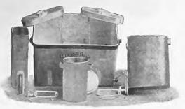
The Separator can be Taken Apart and Put Together in a Moment's Time.
