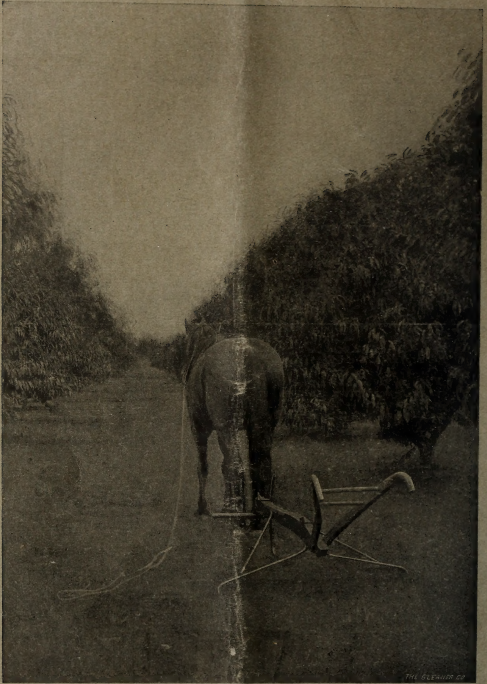
My orchard plow at work in four-year-old orchard. Not patented. Have your blacksmith make one. It leaves a dust mulch. Quickest, cheapest, best.
