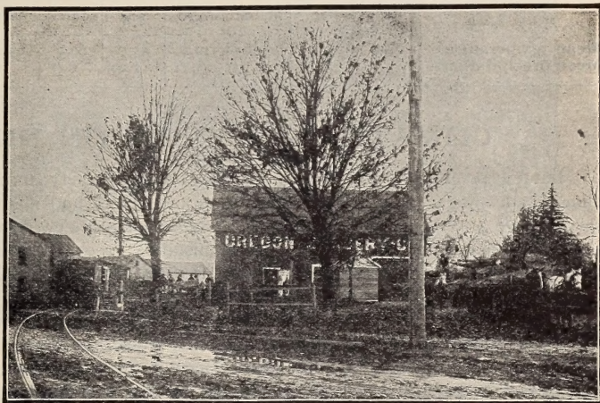
First packing-house, showing building and cars loading on our side-track
