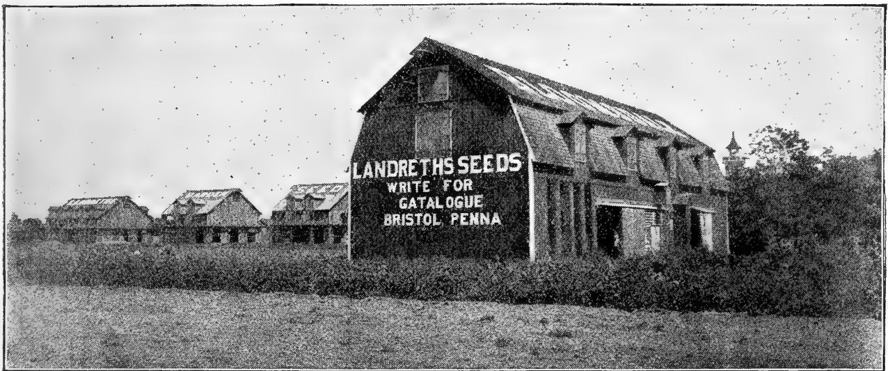
PARTIAL VIEW OF BLOOMSDALE FARM BUILDINGS
