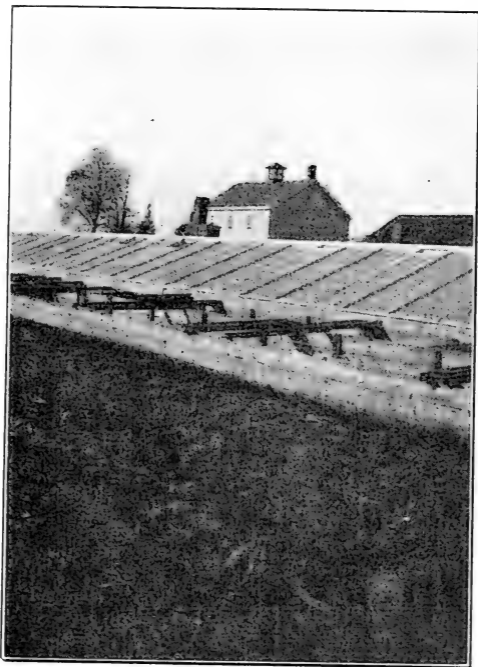
Side view of Mushroom House (formerly a Green House) 162 ft. long by 26 ft. wide. Used the year round for Mushroom Beds.
