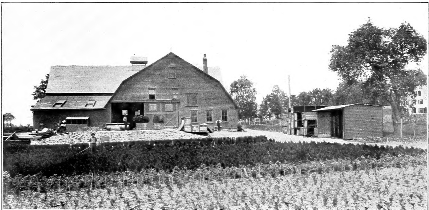
Packing Shed and Platform from which wagons are loaded—Bloodgood Nurseries
