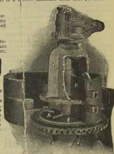
Mechanism of the Mann's showing automatic force feed, cylinder parts, etc. Mann's catalog tells all about it.
