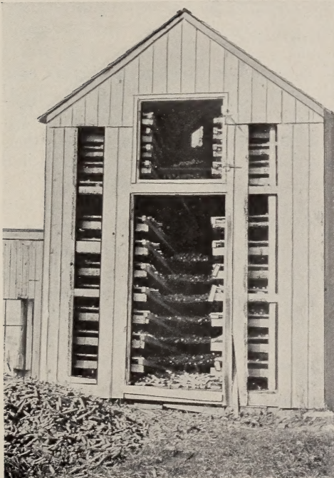
Curing room for Sweet Corn and system of ventilation during late summer.
