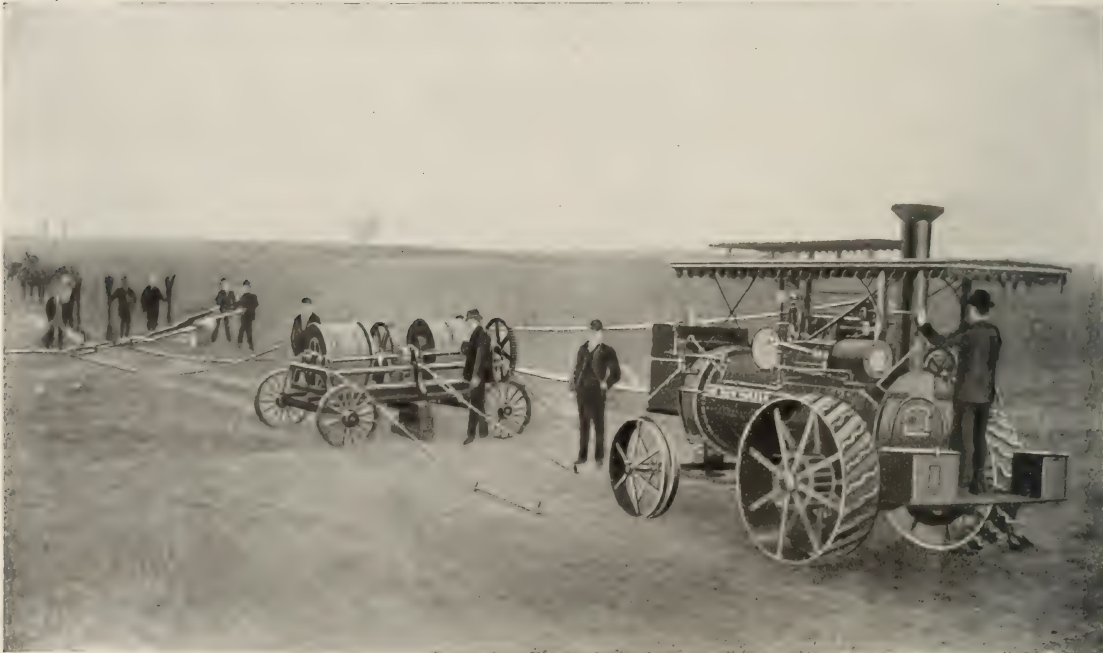
GREENING'S STEAM DIGGER IN OPERATION.
