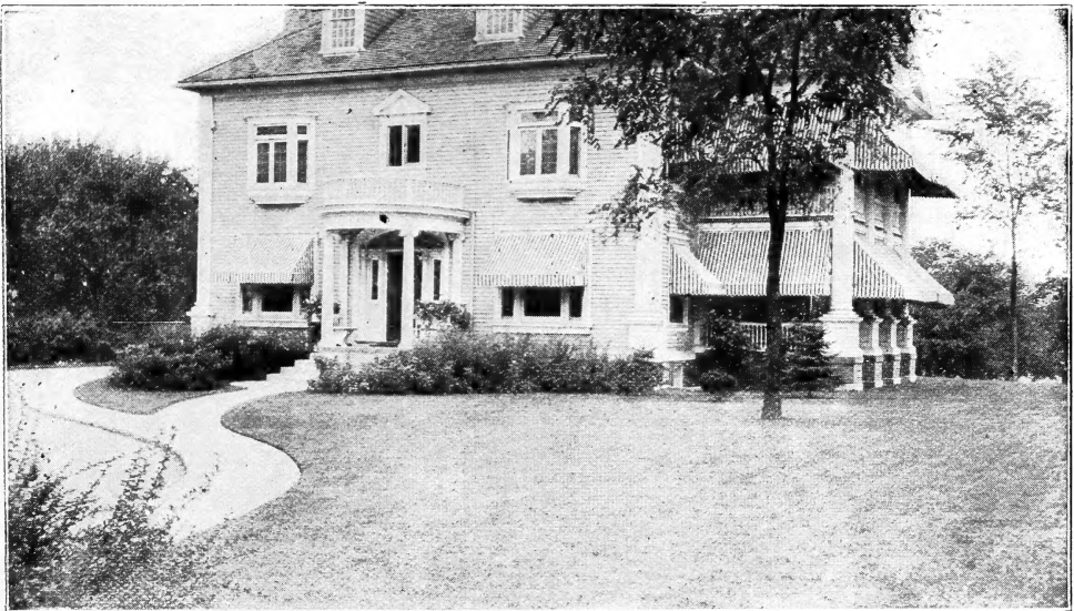
Still another view of open effect in Modern Landscaping.
