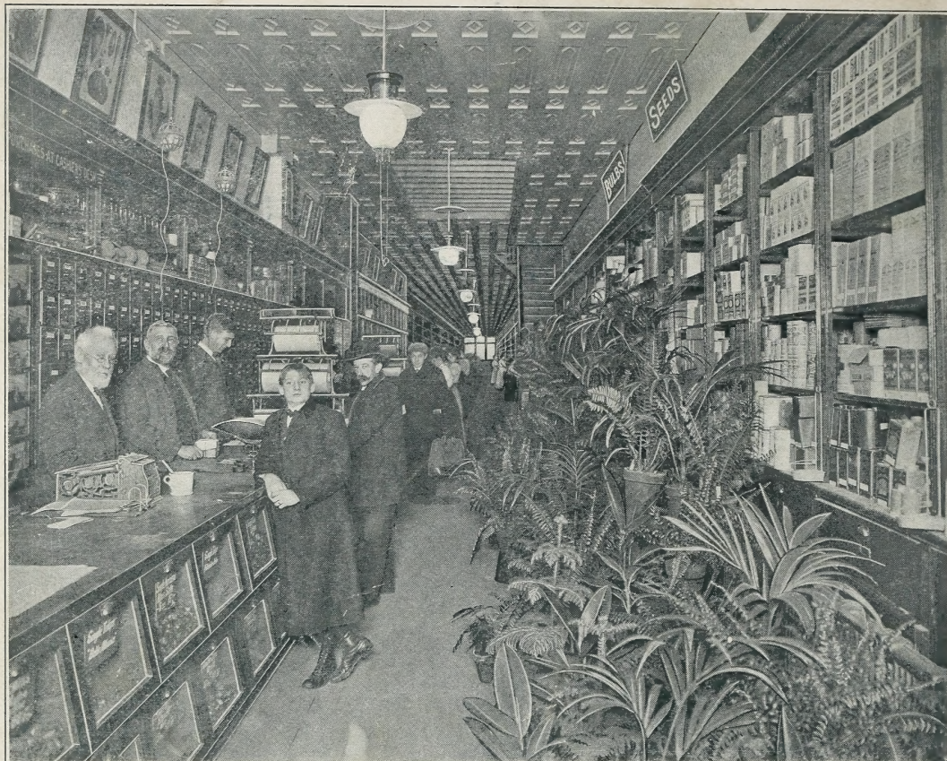
First floor of Johnson's retail store, 217 Market St., extending through to 206 Church St.
