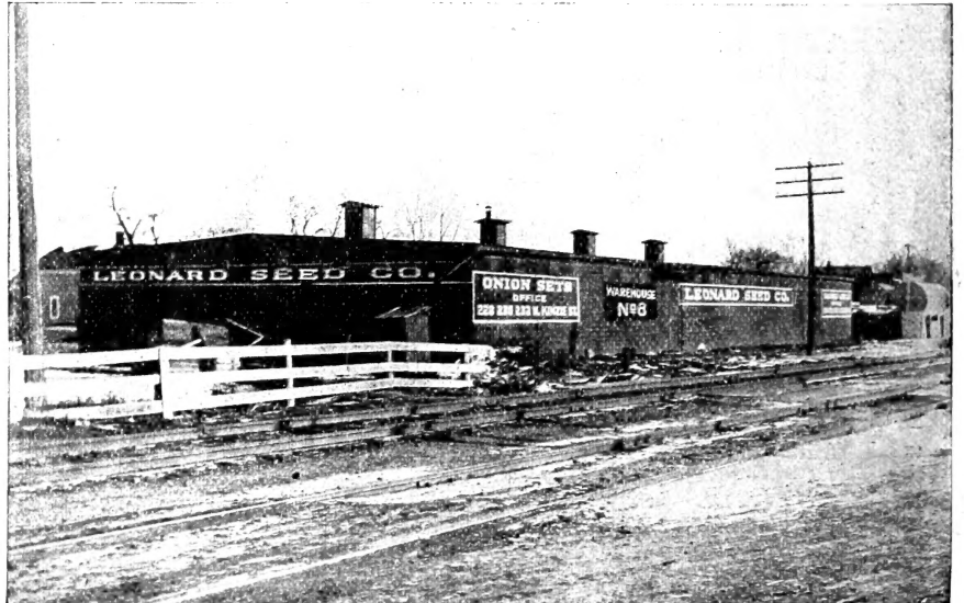
ONION SET WAREHOUSE No. 8 CHICAGO
