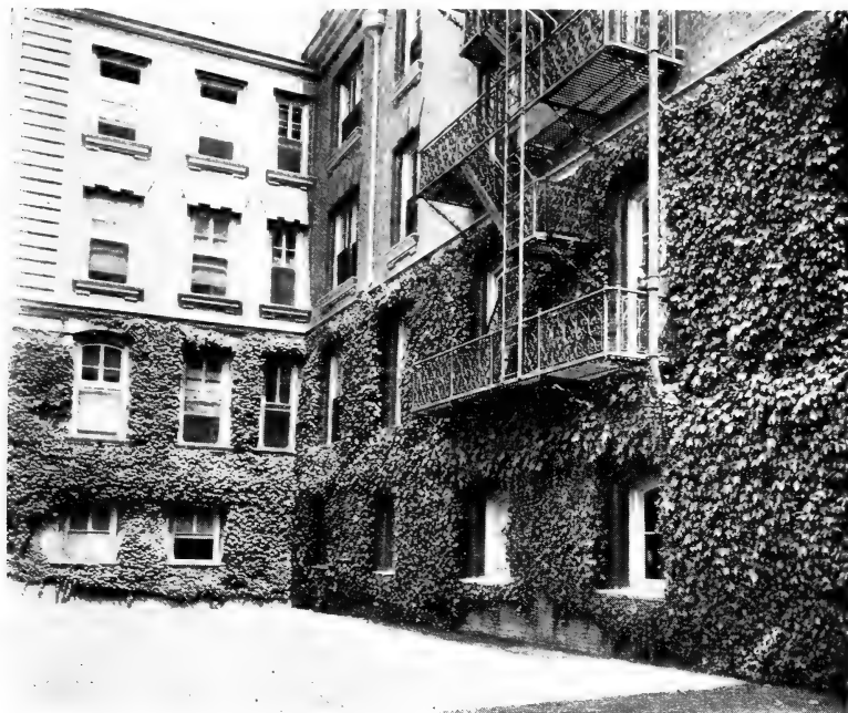
Boston Ivy on Good Samaritan Hospital
