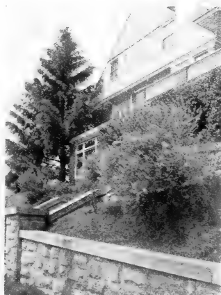
Spanish Broom Vista Avenue
