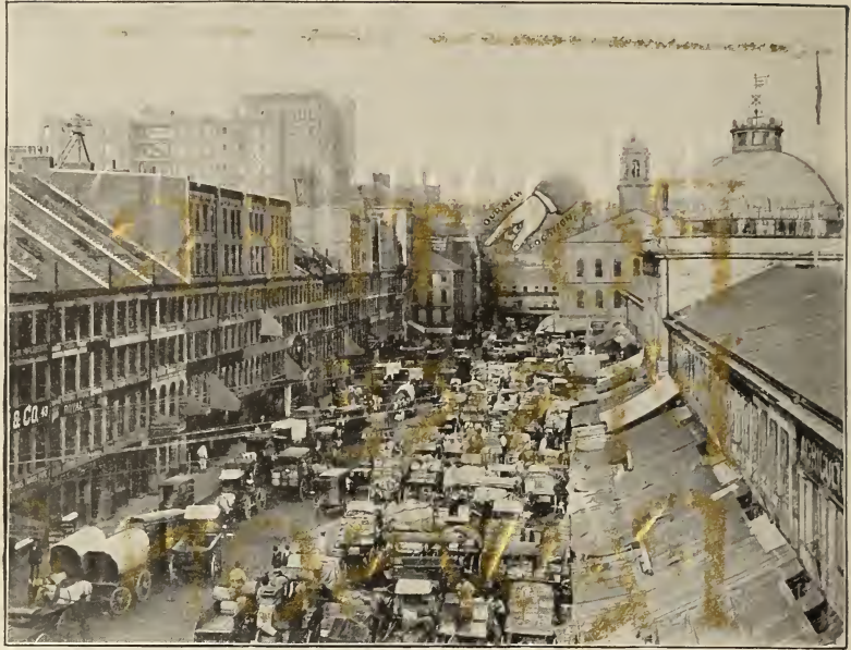
A view of South Market Street taken about 8 o'clock in the morning—just an ordinary busy morning. On the extreme right, just beyond the Quincy Market building, is the "Old Faneuil Hall" and directly opposite is Fottler, Fiske, Rawson Co.'s store just at the head of the market district
