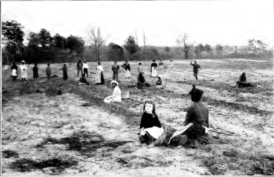
A large force at work on Gandy in April
