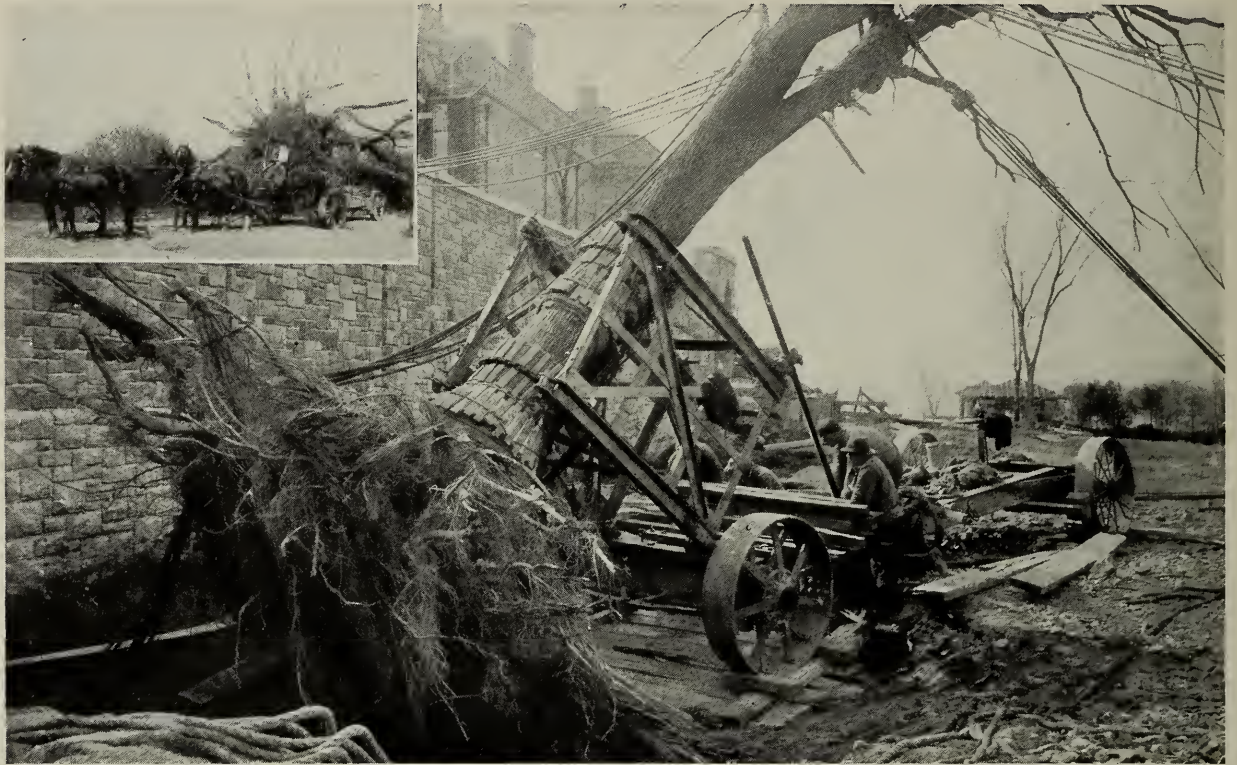
Our all steel mover designed for large deciduous trees. With this we can move trees 70 ft. high, 50 ft. wide, with an area of roots 45 ft. in diameter. The illustration shows an Elm being moved. Note how the tree rests in the steel cradle, padded to distribute the pressure. Two screws swing the tree over.
