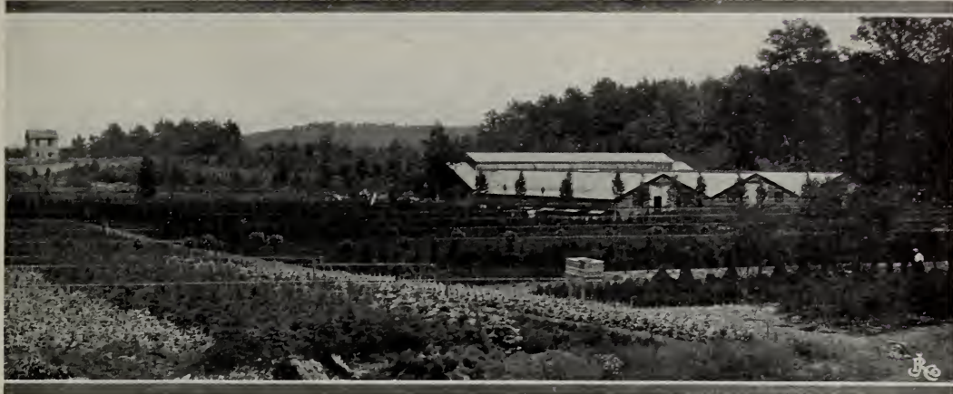
A Partial View of Our Nurseries, Showing Storage Sheds in Background
