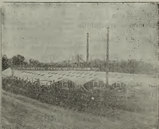
Partial View of Our Greenhouse Plant.
