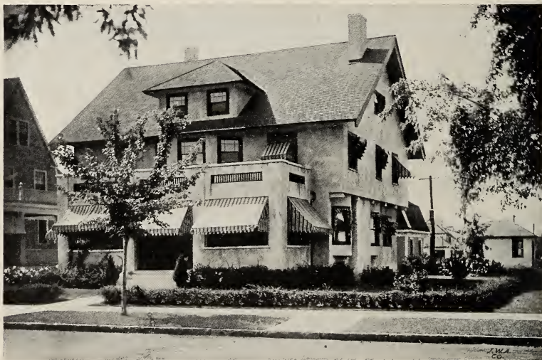
Result Obtained Six Months after Building was Completed
