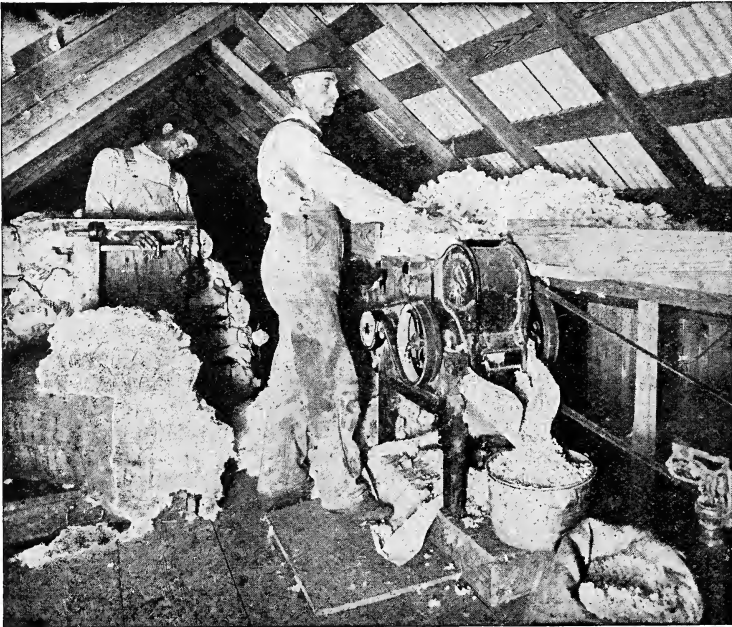
Laboratory Gin—10 saws.—Used in ginning individual stalk selections and in making accurate determinations of the per cent of lint in the harvest from progeny rows, multiplying blocks, and to keep our stock seeds free from any mixing.
