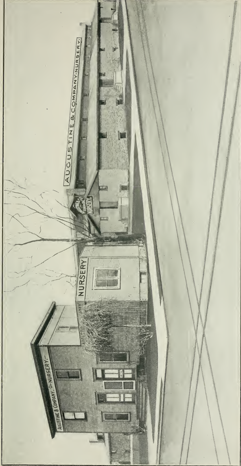
Our new packing house, just completed, giving us 12500 square feet of floor space with every modern convenience.
