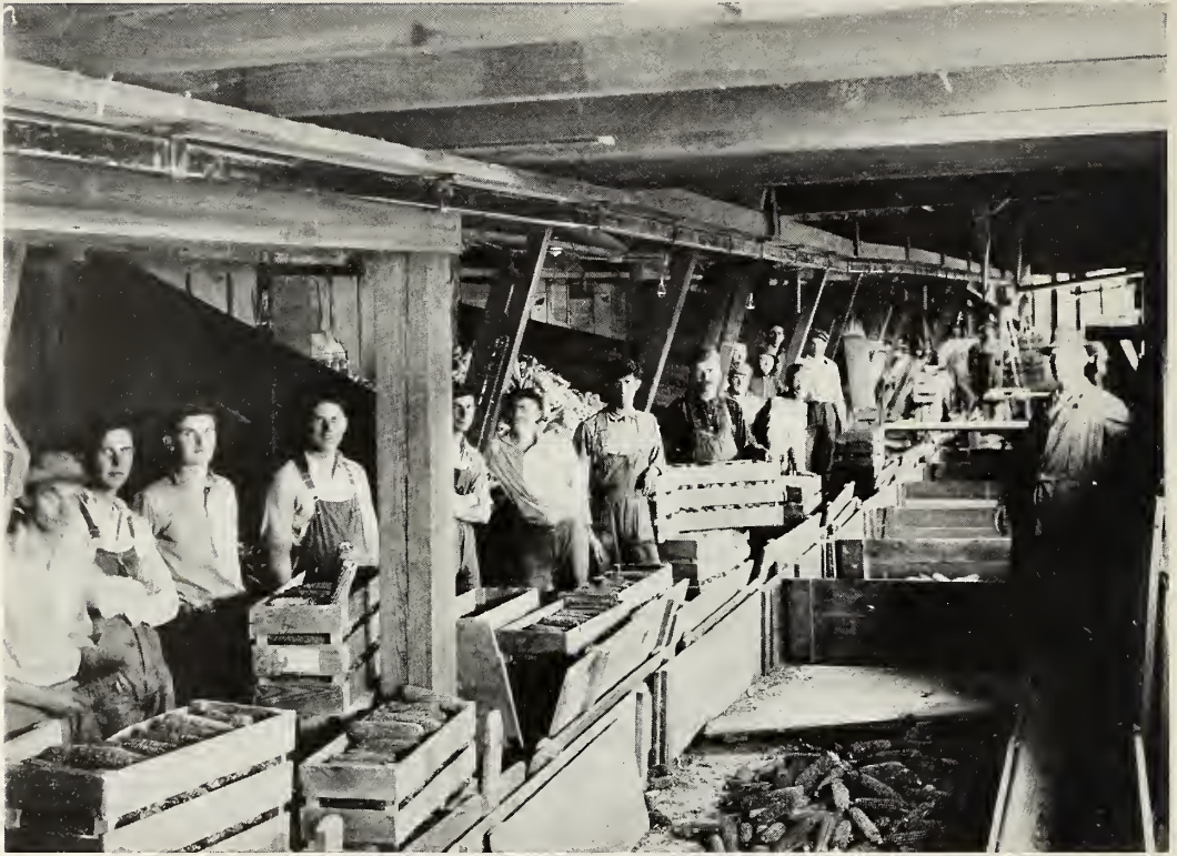
SORTING ROOM IN BASEMENT
