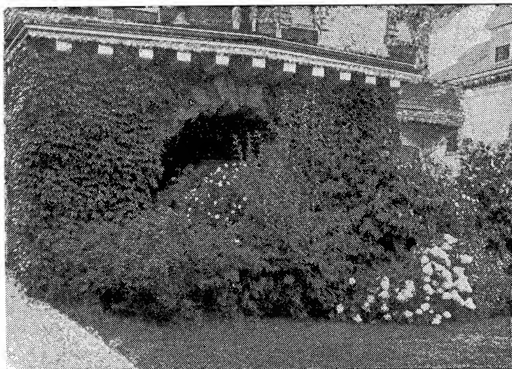
Ornamental plantings are much desired at the house foundation. At a trifling cost, the owner of this house increased its beauty a hundredfold
