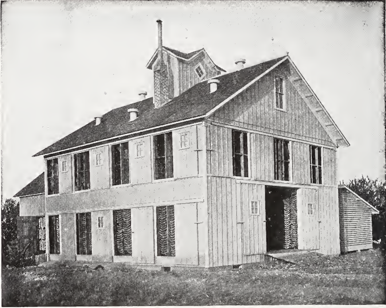
Dry House, showing doors opened for a nice, warm day. Notice perfect ventilation through the doors, allowing the air to pass on through the ventilators in the roof
