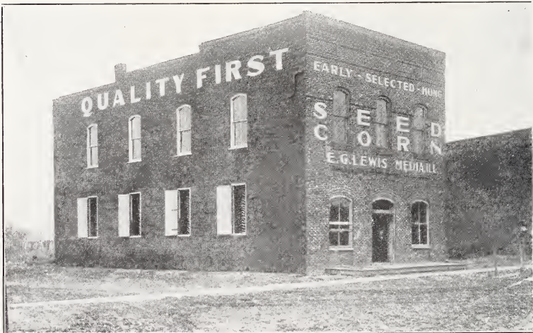
The lower story of this building has a capacity of 2,000 bushels for Hung Seed Corn. It is also equipped with a large hot air furnace.
