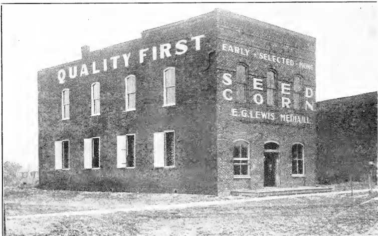
The lower story of this building has a capacity of 2,000 bushels for Hung Seed Corn. It is also equipped with a large hot air furnace.
