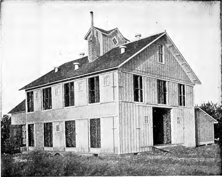
Dry House, showing doors opened for a nice, warm day. Notice perfect ventilation through the doors, allowing the air to pass on through the ventilators in the roof
