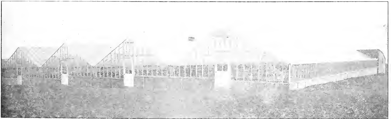
A part of our Greenhouses at Olive and Price Roads. These houses are 25 feet wide and 100 feet long, of concrete and steel-frame construction.
