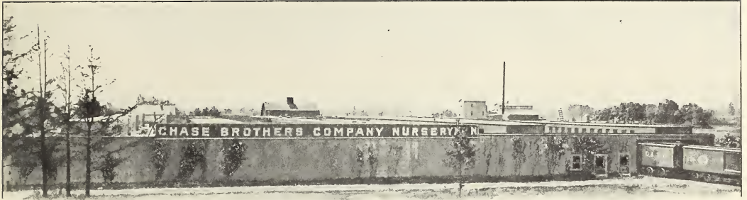
Our Packing Cellars are thoroughly modern and built for the purpose
